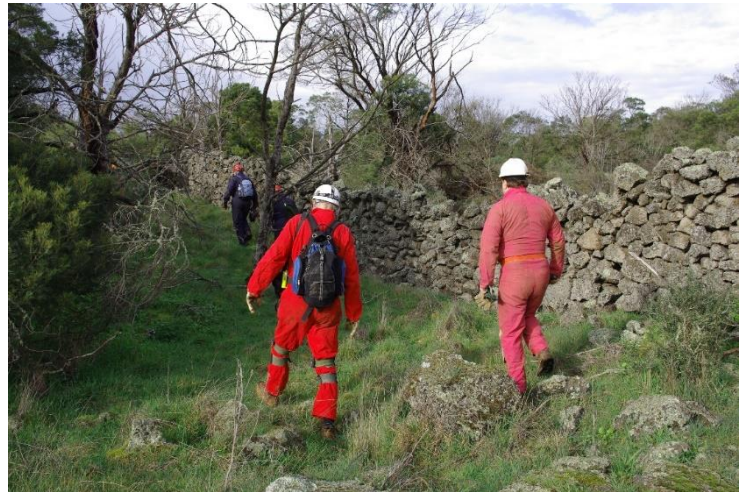
Figure 7. Typical dry stone wall fashioned from loose blocks of basalt.
