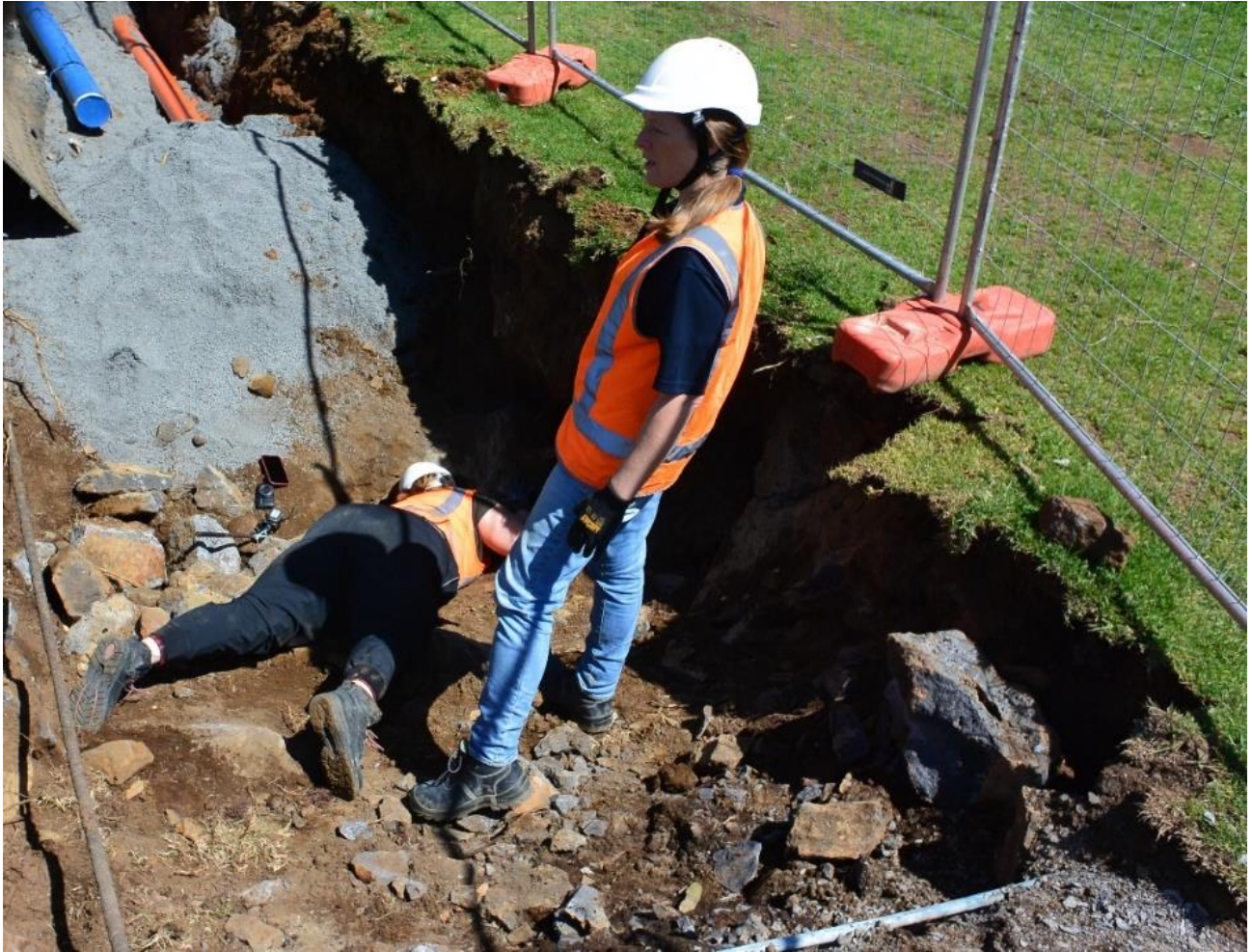
Figure 19. Temporary access point to a small void discovered during pipeline work in Roosevelt Ave.
