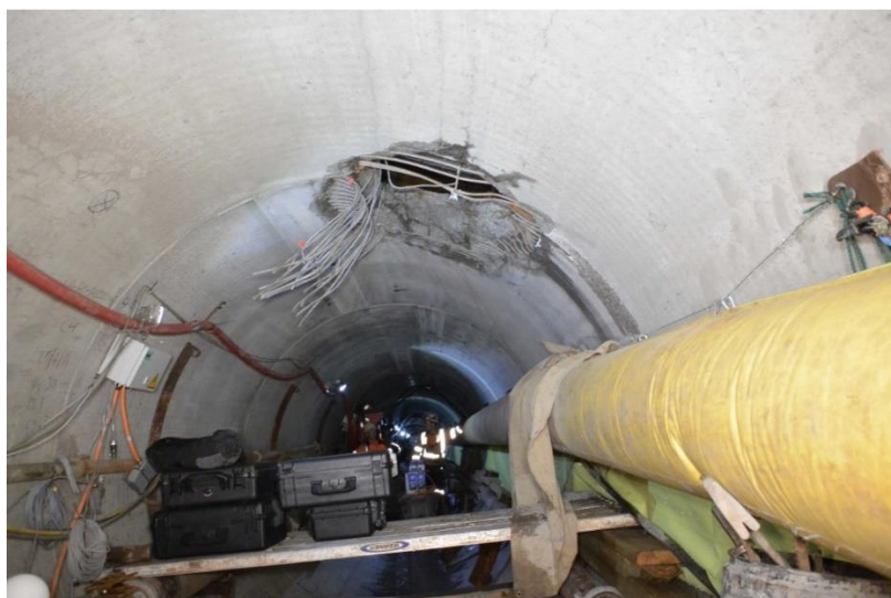
Figure 12. A view from inside the damaged concrete lining of the Hunua Tunnel. The hole was created while the pipe was being pushed along the tunnel. The hole has been enlarged to facilitate inspection, assessment and repair work.
