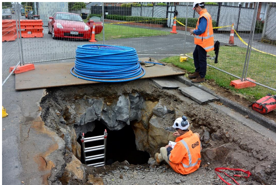
Figure 7. The cave passage revealed by an exploratory hole dug in Ngatiawa Street after preliminary investigations suggested a high likelihood of a cavity.
