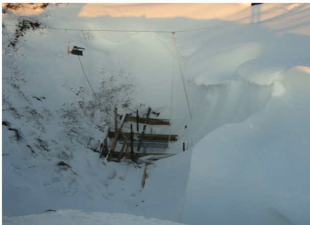
Fig. 8. The entrance depression partially filled with snow and the working platform destroyed — a minor setback.
