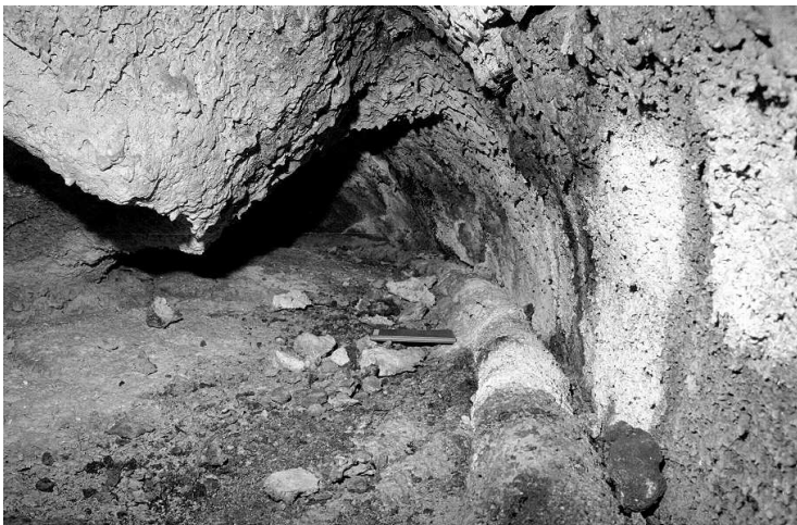
Figure 5: Looking south from section X4. Note the small rolled bench against the foot of the wall and the pale patches on the wall. Notebook is 18 cm long.
