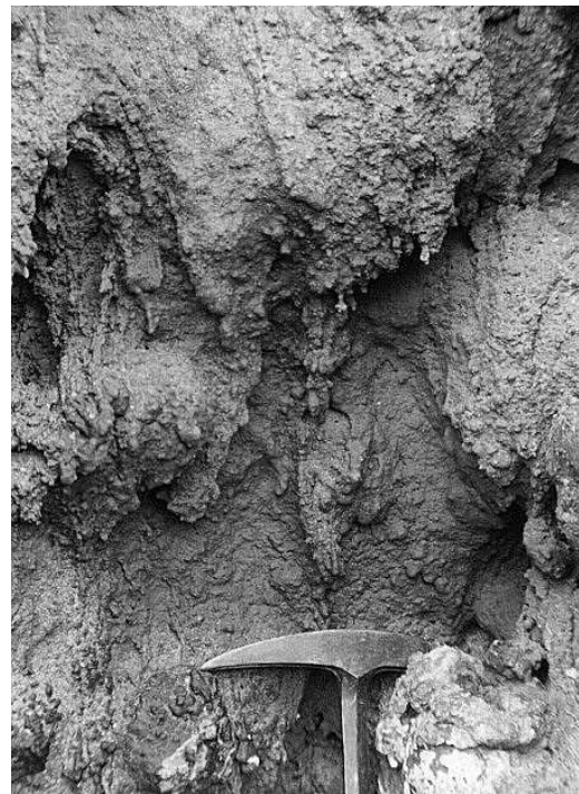
Figure 6: Spatter and drips in a vertical pipe.
