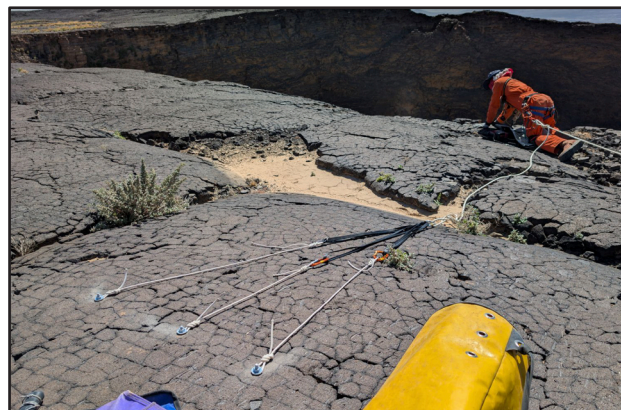
fig. 12: Use of dyneema, Korda's Rope and long M10 anchors in fractured Pāhoehoe lava; picture by R. Haemers
