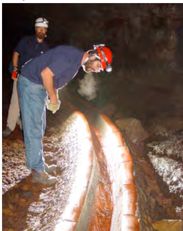
Fig. 26. Ceramic-lined trench, Furna d'Água, Terceira
